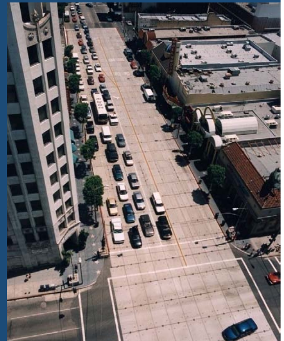
Concrete decking along Hollywood Blvd. during Red Line Construction
