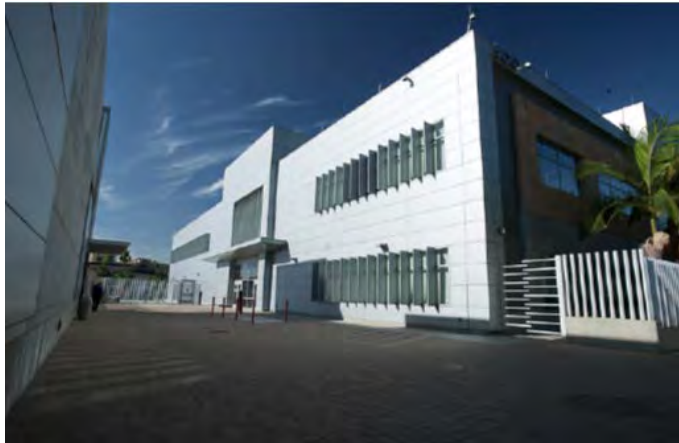
City of Los Angeles EOC
