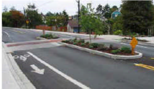
Class II Bicycle Lane (Dedicated On-Street)
