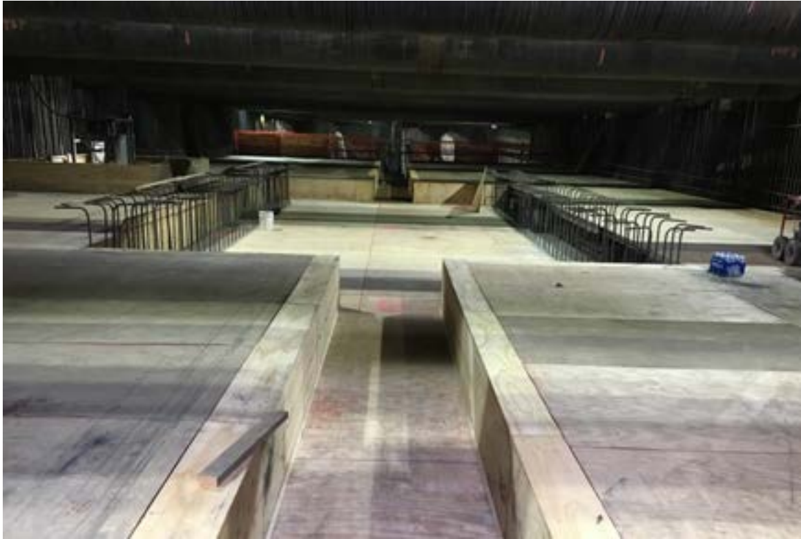
Concourse deck construction inside Wilshire/La Brea Station.
