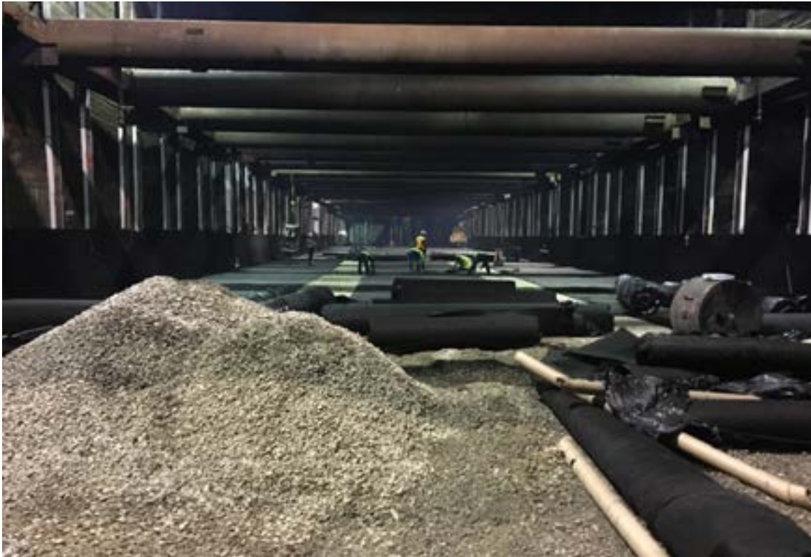
Buidling the floor inside the Wilshire/Fairfax Station.
