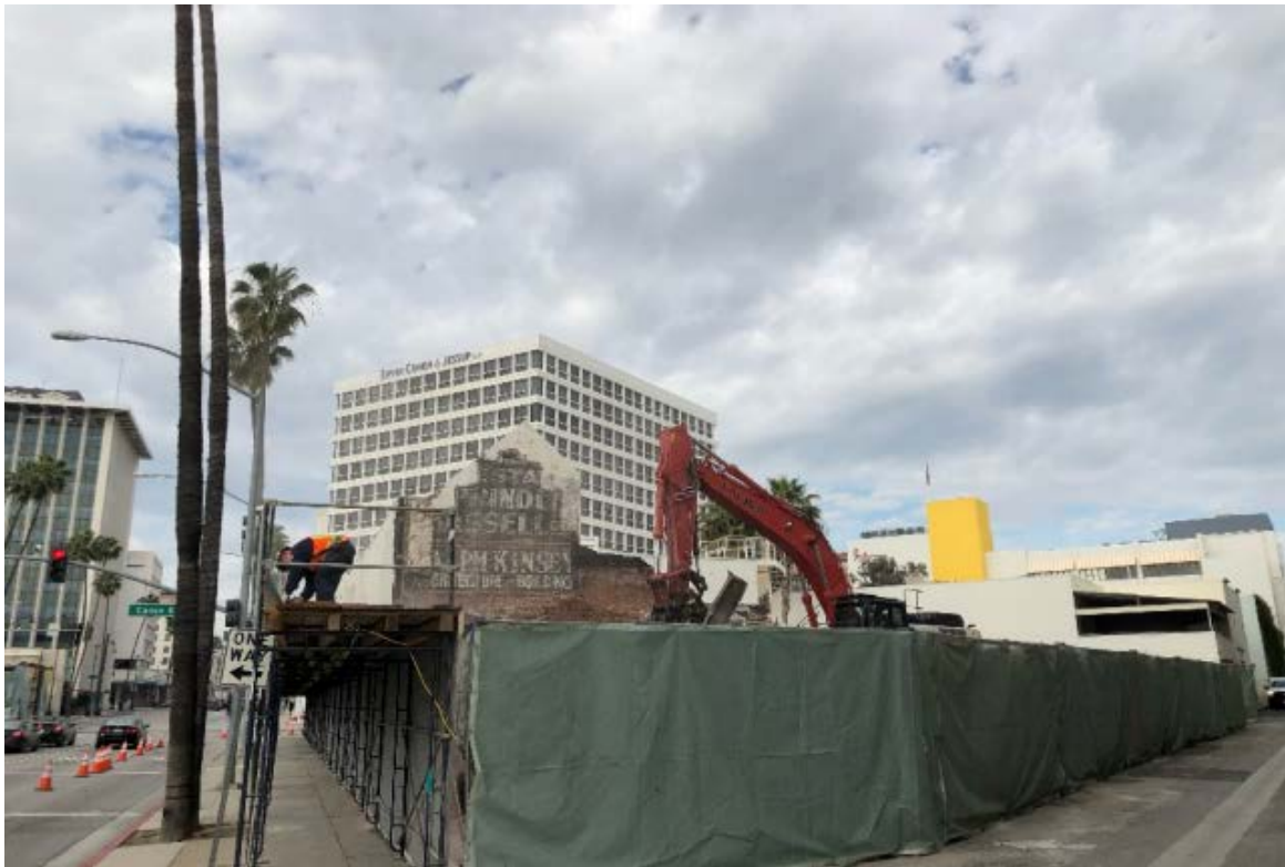
N. Canon properties demolition progress.
