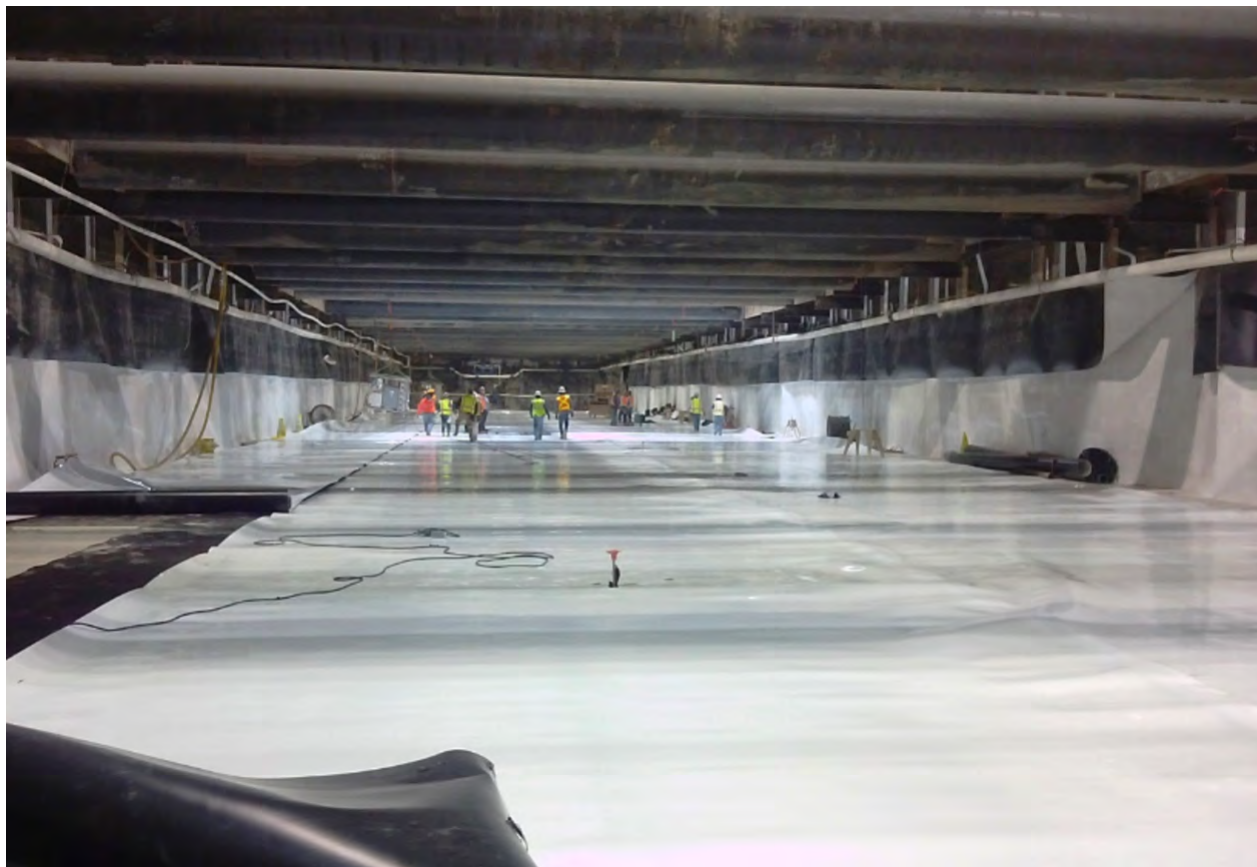
Caption: Installing the HDPE layer inside Wilshire/La Brea station
