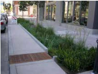
Examples of stormwater infiltration treatments
