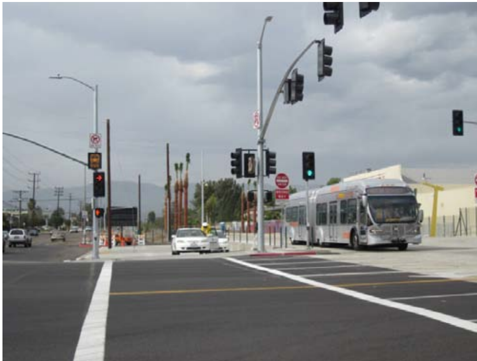
Bus testing on alignment.
