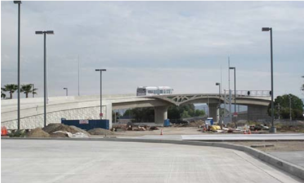
Bus testing over Lassen Bridge.
