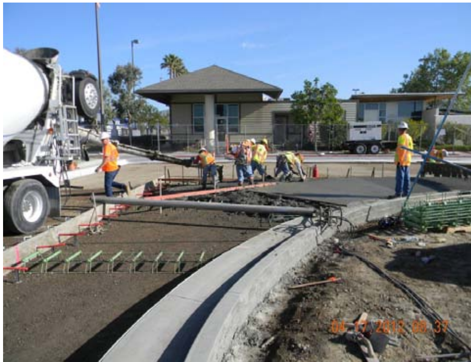
Paving at Chatsworth Station.
