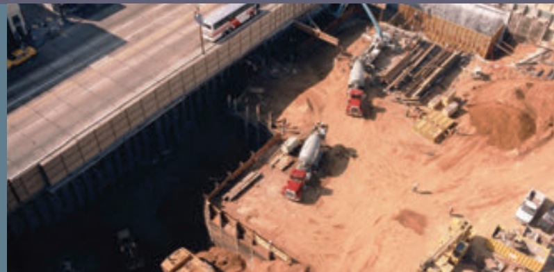
Staging for the Hollywood/Highland Station during construction of the Metro Red Line. Note traffic continuing to flow on Hollywood Bl.
