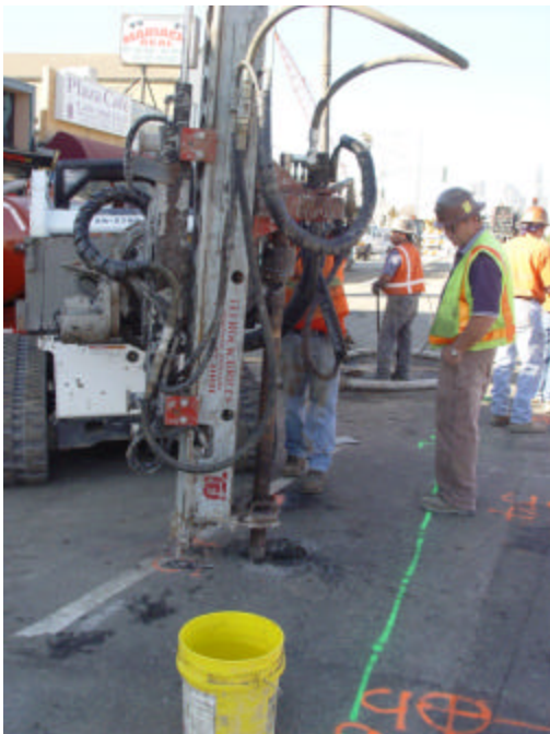
Drilling and grouting at 1 st Street and Boyle Avenue
