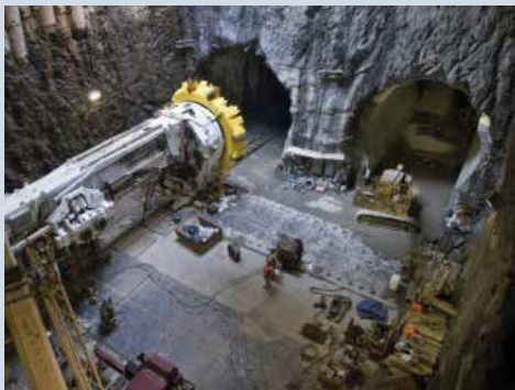
J.F. Tunneling Activity for New York's 2nd Avenue Project
