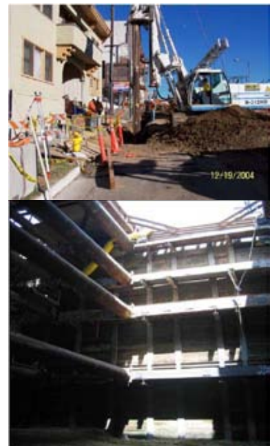
Figure 2-2. Typical Cut and Cover Construction Activities
