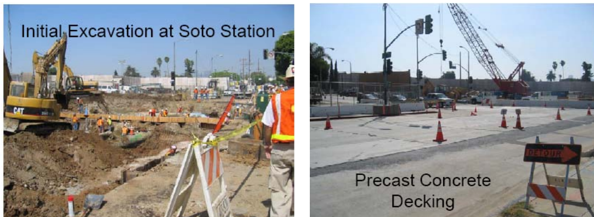
Figure 2-2. Typical Cut and Cover Construction Activities
