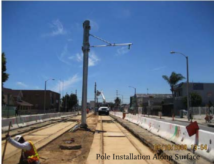
Figure 3-4. Typical Drilling and Installation of Pole
