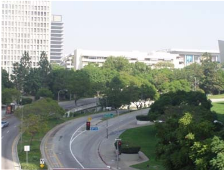
Figure 4-11. Open Space at West End of 2 nd and 3 rd Street Tunnels
