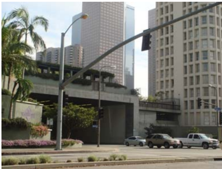
Figure 4-12. West End of 2 nd Street Tunnel
