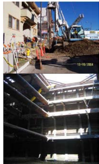
Figure 2-2. Typical Cut and Cover Construction Activities
