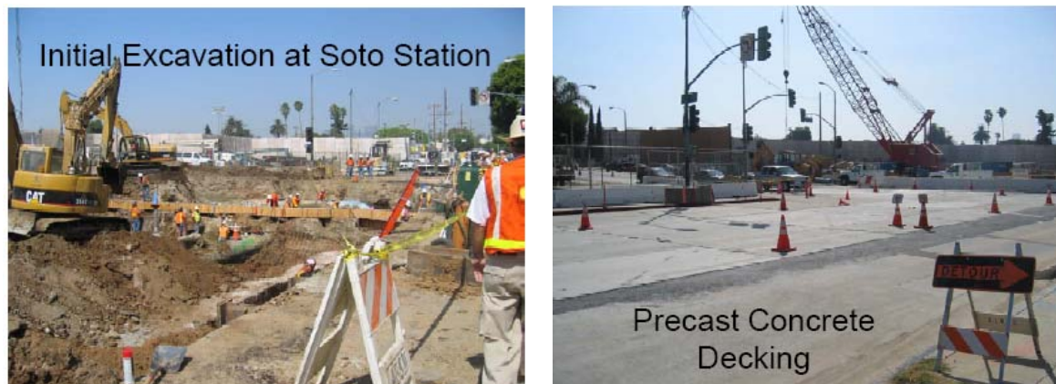
Figure 2-2. Typical Cut and Cover Construction Activities
