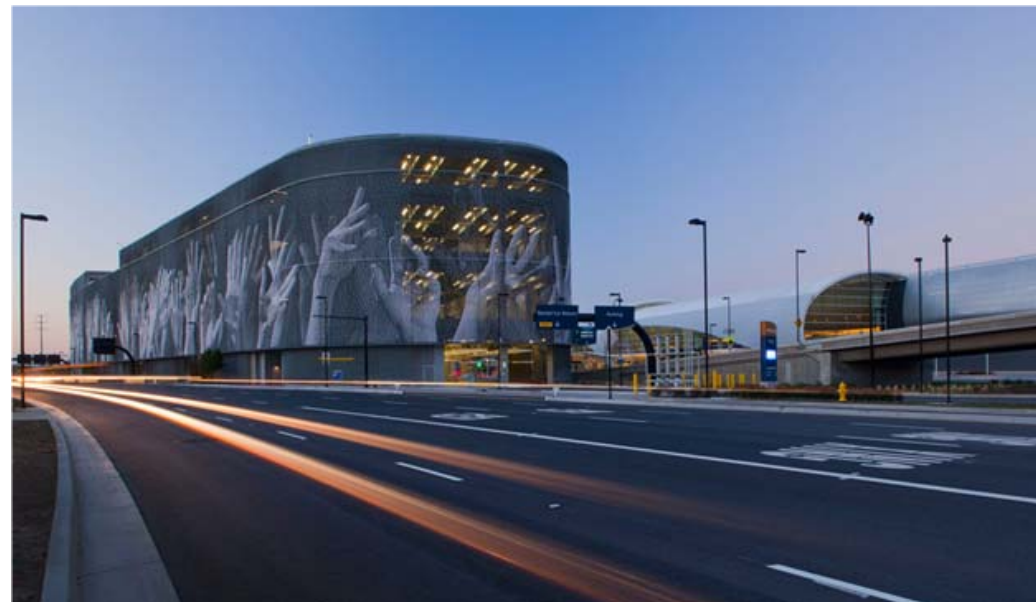
San Jose International Airport ConRAC
