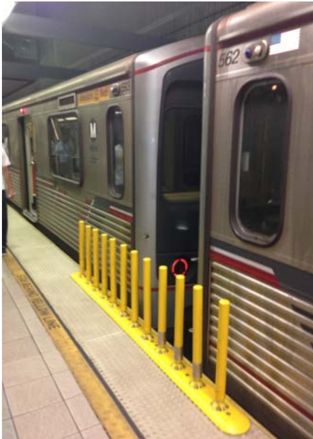
Between Car Barriers & Tactile Warning Strip
