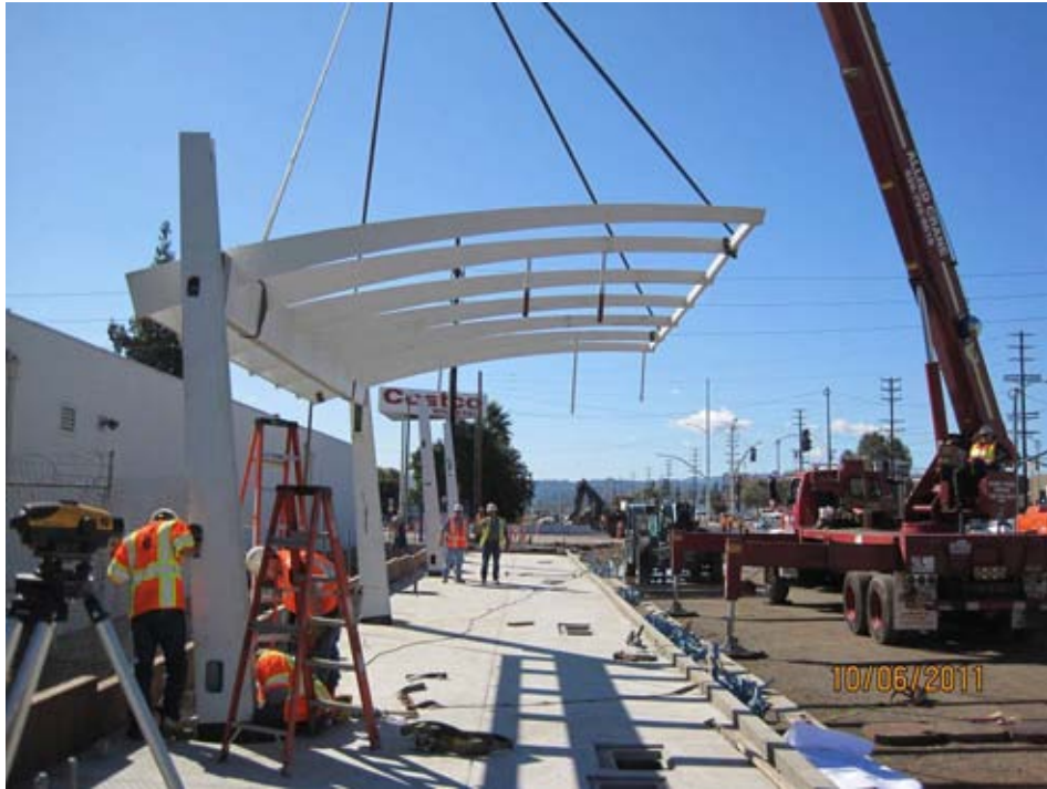
Placing canopy at Roscoe Station.
