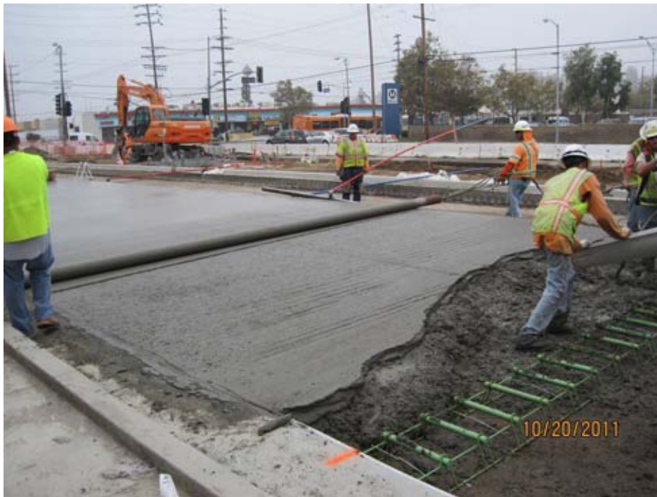
Placing busway pavement at Nordoff.
