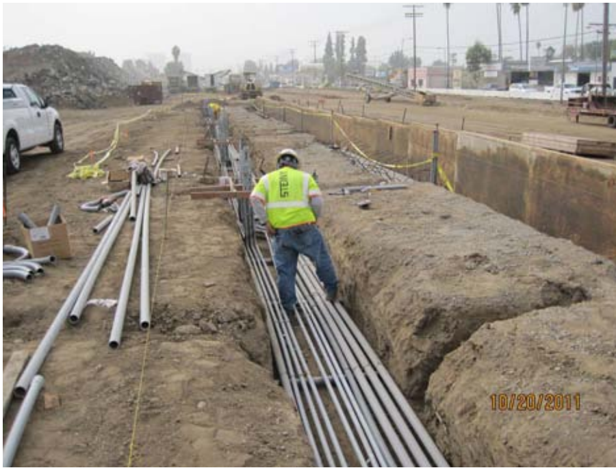
Placing ductbank at Sherman Way Station.
