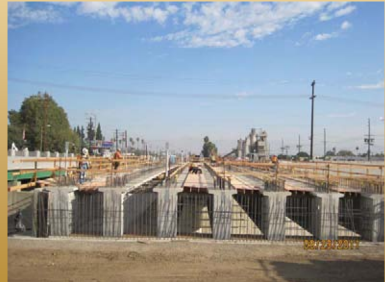
Forming Deck – LA River Bridge
