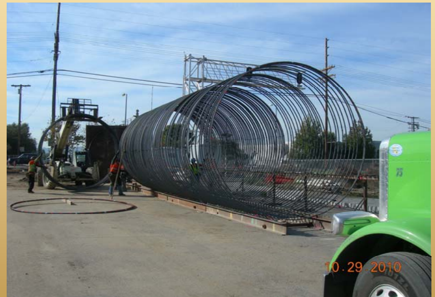
Rebar for large diameter shaft foundation for Bent 3 of Lassen bridge
