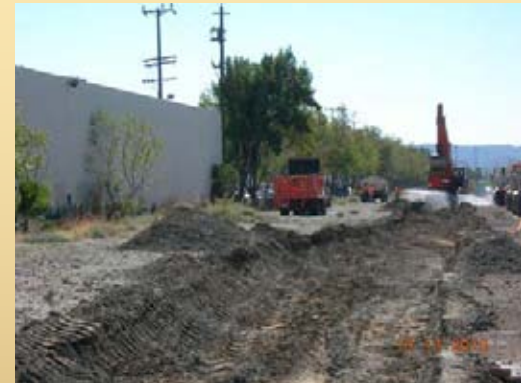
Excavation and removal of soils in proposed busway
