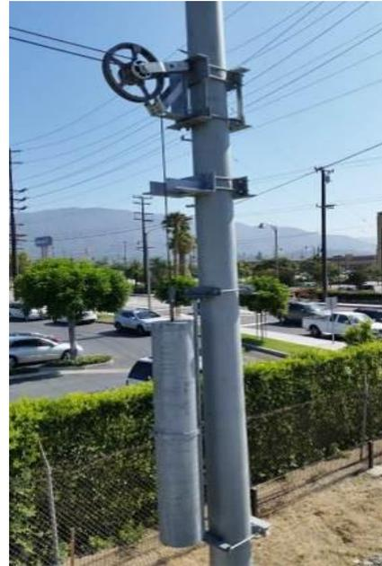
**Figure 15: Existing weight stack tensioning system**
