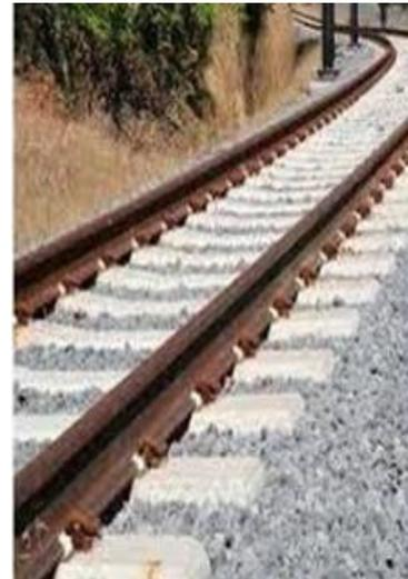
**Figure 7: Concrete sleepers prevent deformation in rail**
