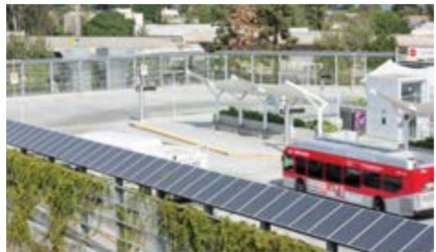
Figure 2-1 Solar Panels at El Monte Station.
