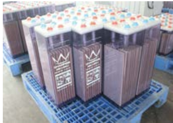
Figure 4-5 A Lithium-ion battery bank similar in size can be expected at typical Metro stations.
