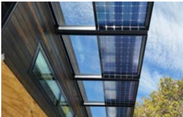
Figure 3-1 Combination of framed bifacial solar panels and glass panels within a framed assembly, French Laundry Restaurant, Yountville, CA.
